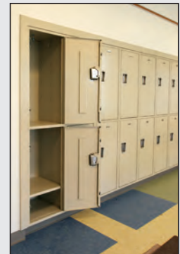
ADA locker has shelf at least 15 inches from floor.
