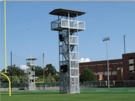
Prefabricated Sports Video & Viewing towers provide coaches and videographers a safe and secure way to observe and film team practices. Our prefabricated, sectional, design facilitates quick and easy construction to minimize impact to on field activities.
