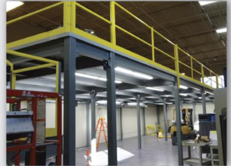
Mezzanines: Storage Platforms, Equipment Platforms, Conveyor Crossovers and Fall Protection Platforms. Heavy-duty structural steel components designed in accordance to IBC building code.
